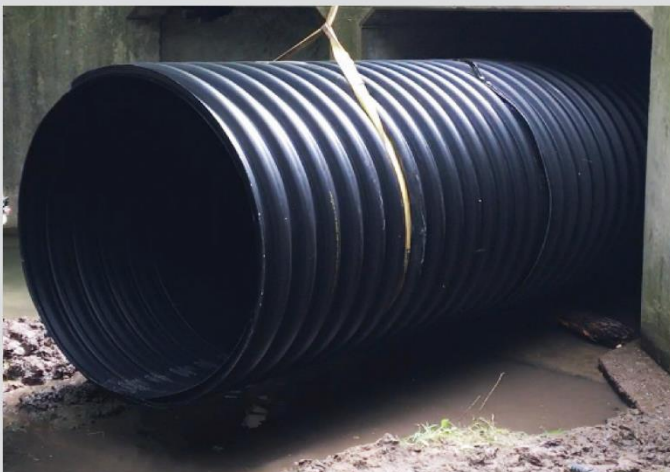
Iowa 72" pipe slip, two runs, 83' lengths
